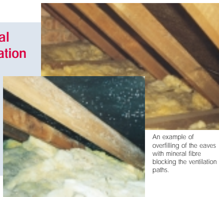
An example of condensation and mould growth.
