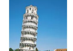
042 Leaning tower of Pisa, Italy
